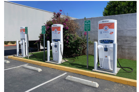
Tritium 50kW fast chargers on the EVCS network
